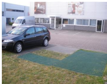
Afb. 2: Direct na montage
